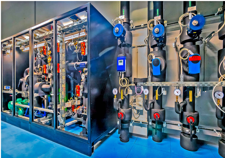
View of pipes that form part of the water-cooling technology of the Lenovo NeXtScale systems.
