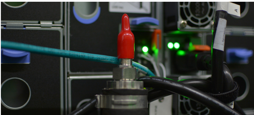
Close-up view of pipe that forms part of the system’s direct water-cooling design.
