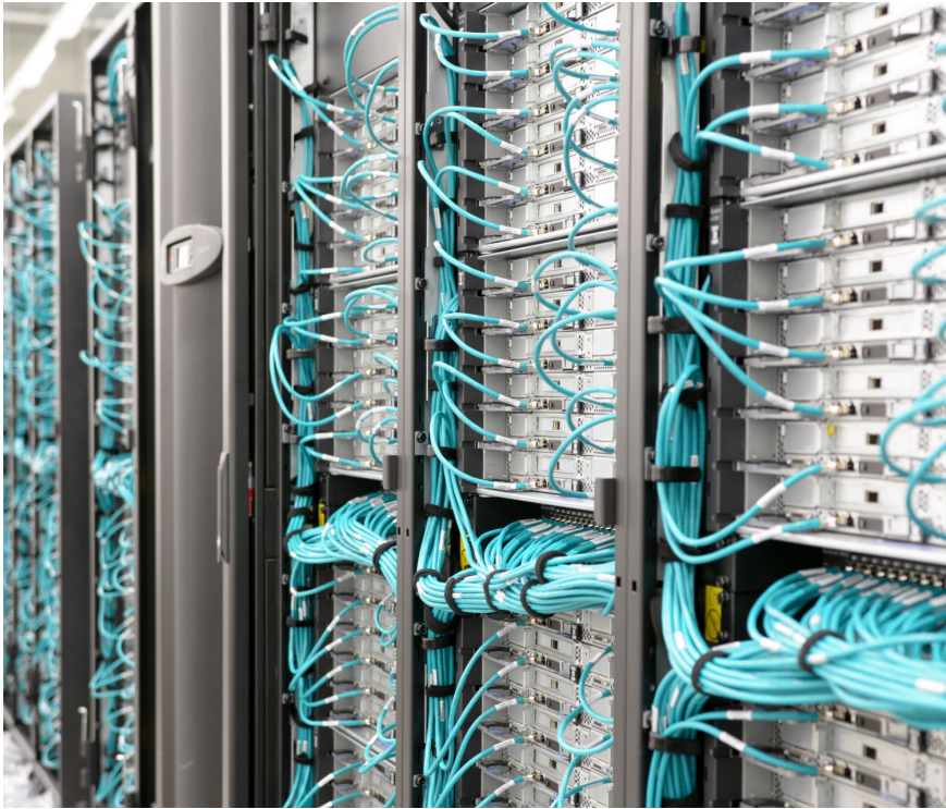
View of SuperMUC Phase 2 powered by Lenovo NeXtScale systems.
