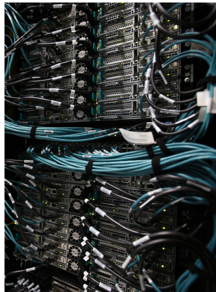
Close up of Lenovo NeXtScale System M5.
